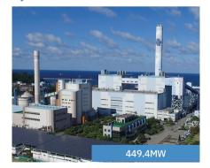
The Donghae Power Complex is a fluidized bed power plant that uses anthracite produced in Gangwon-do as a power generation fuel. It contributes to maintaining the local coal mining industry, and recently, it has initiated the operation of a biomass power plant that uses abundant local waste wood as fuel, thus building an ecosystem for the related industry.
