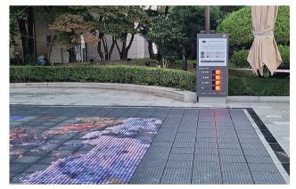
Application of "pavement block solar power"
