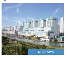
The Dangjin Power Complex serves as EWP's core power plant, playing a pivotal role in the power supply in the central region of Korea. It pursues pollutant minimization in the process of power generation, such as pollution control facility improvement projects, including the replacement of the flue-gas desulfurization (FGD), deNOx system, and adding indoor coal storage to reduce fugitive dust.
